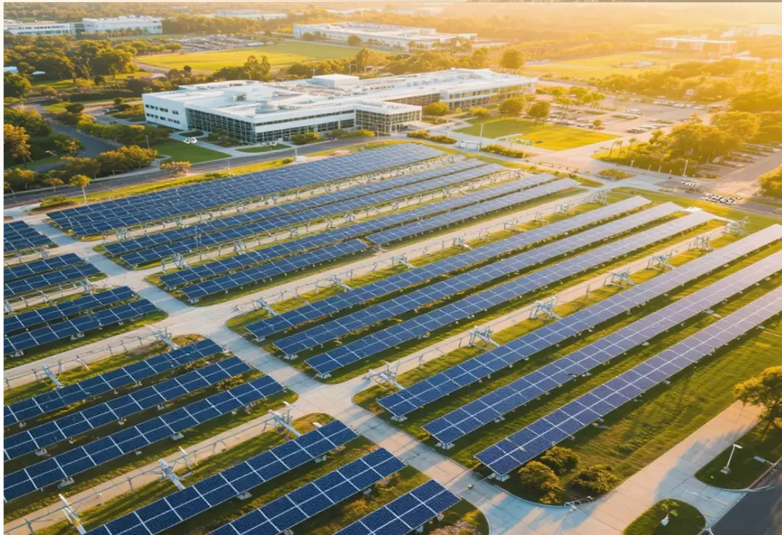
PV-Storage-Hydrogen at Google's Silicon Valley Campus
